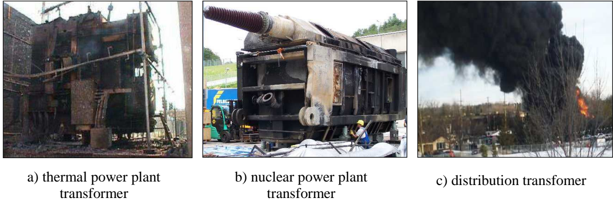
Figure 1 – Transformers explosion examples
